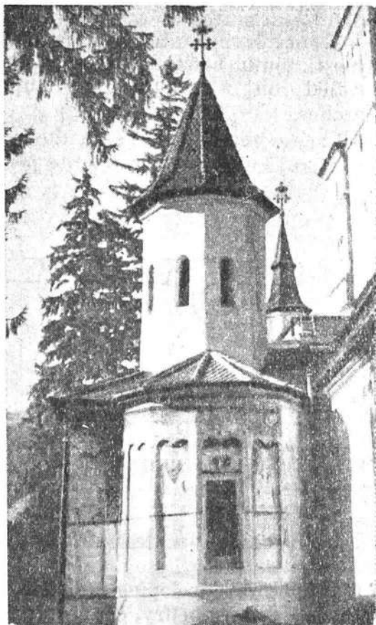
Fig. 32. — St. Nicholas church in Șchei Brașovului. The southern chapel seen from the East.
