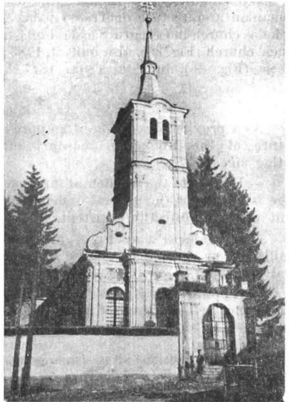
Fig. 36. — St. Nicholas church in Baciu—Săcele. Western façade.
